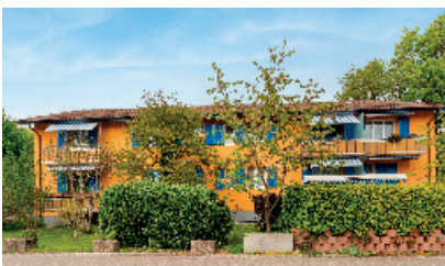
Wallisellen Alte Winterthurerstrasse 104, 106
